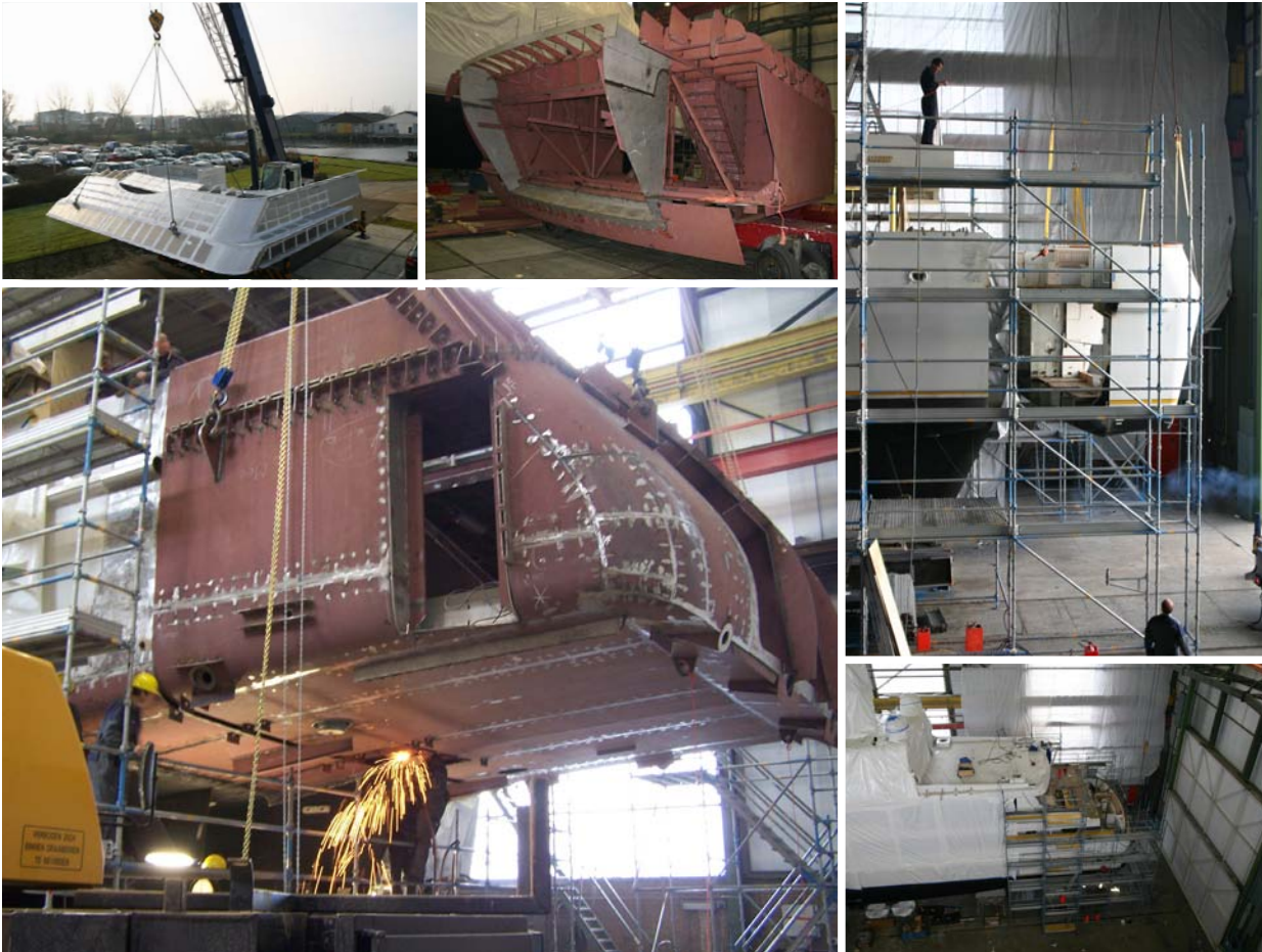
The original White Rabbit carried an impressive array of toys, but was significantly reconfigured during the refit. A 1.75m section of her stern was cut off and a new 5.25m stern section was added, extending the LOA by nearly three metres. More impressive, though, is the resulting increase in deck space with all decks being extended. Pegasus now features 265 square metres of outdoor entertaining areas
